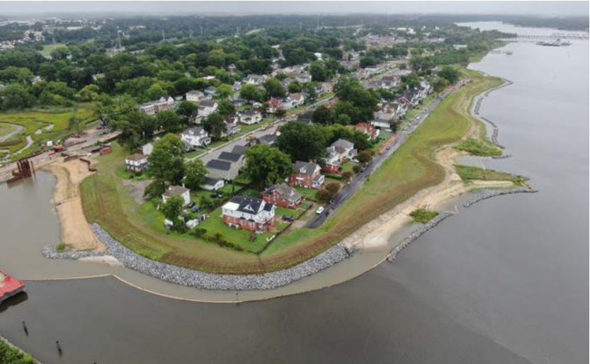
Aerial photo of living shoreline and berm under-construction
